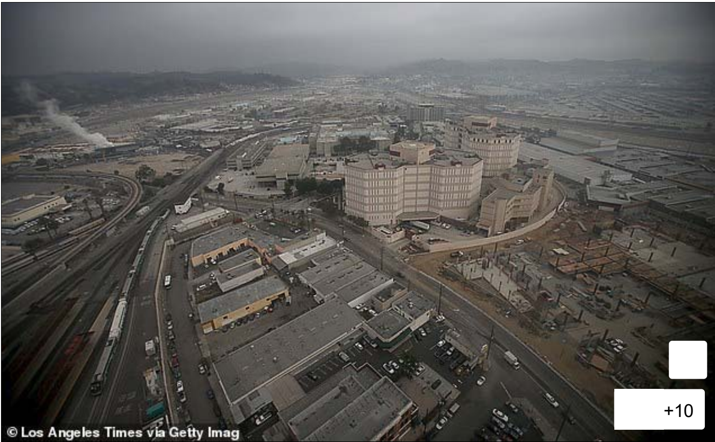
The Los Angeles River flows behind the Twin Towers Jail in Los Angeles County. Five inmates are in quarantine in the correctional facility as a result of the coronavirus
