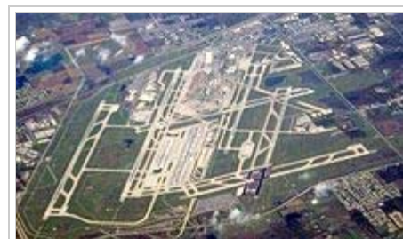
An aerial view of Detroit Metropolitan Wayne County Airport
