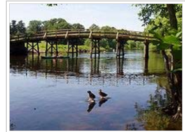
The reconstructed North Bridge in Minute Man National Historical Park, Concord
