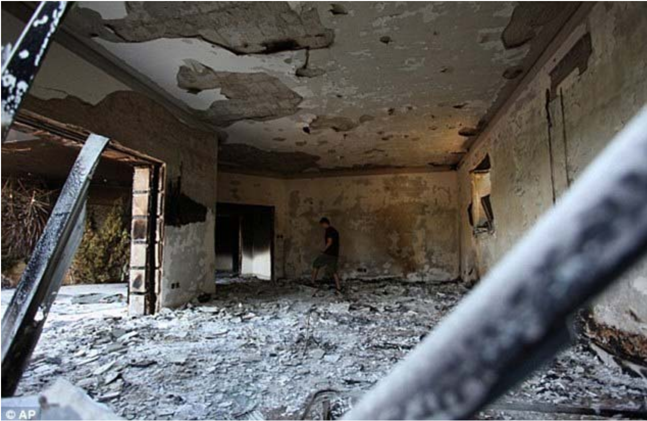
Inferno: Armed attackers dumped cans of diesel fuel and set ablaze the consulate's exterior
