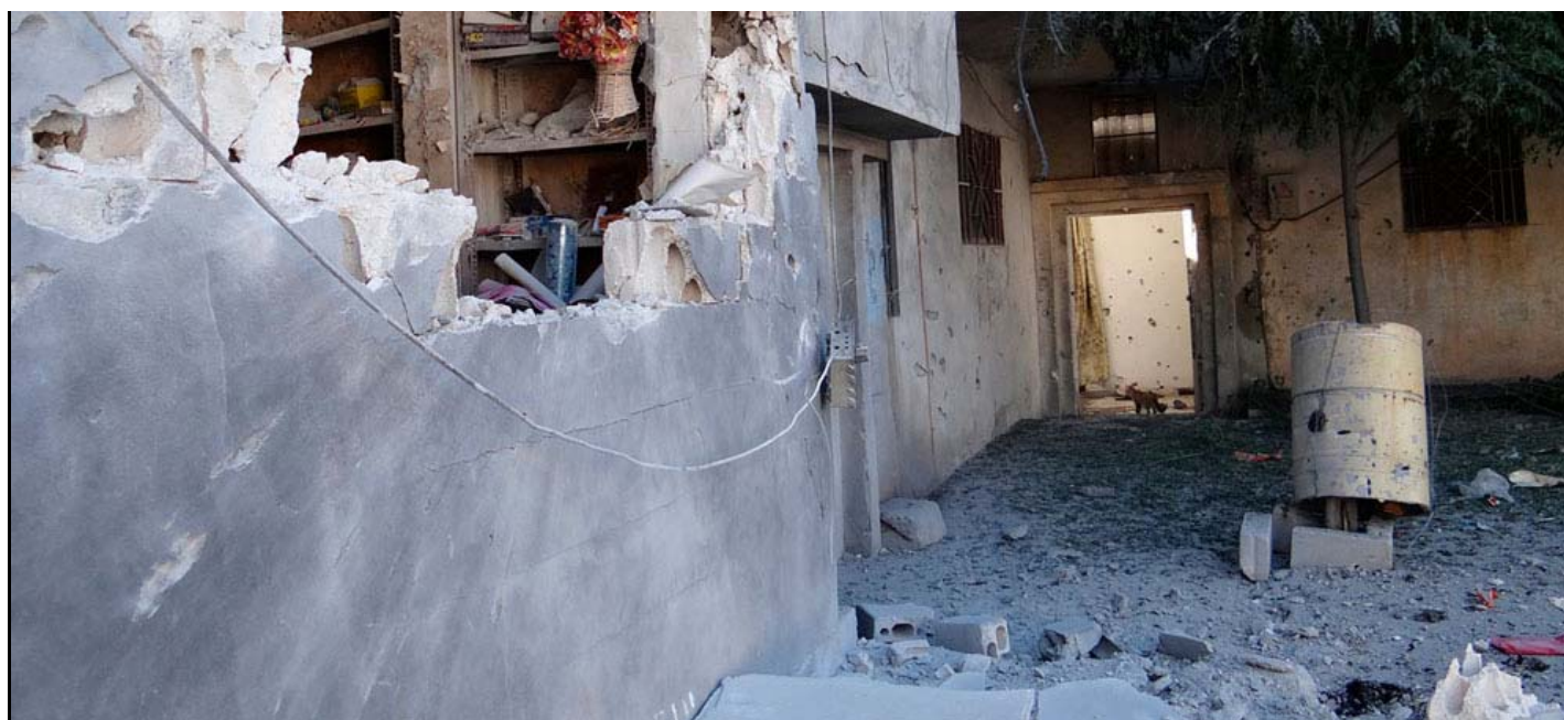
34 A damaged building, after shelling of the Talbisah area in Homs city, on June 13, 2012. (Reuters/Sham News Network) # □
