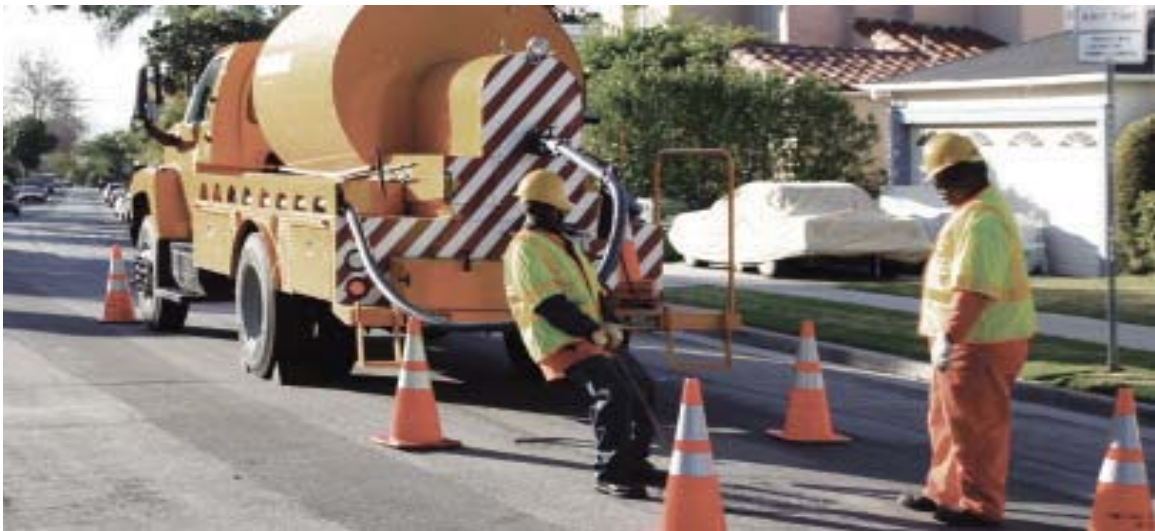
Los Angeles operates and maintains the largest wastewater collection system in the United States.
