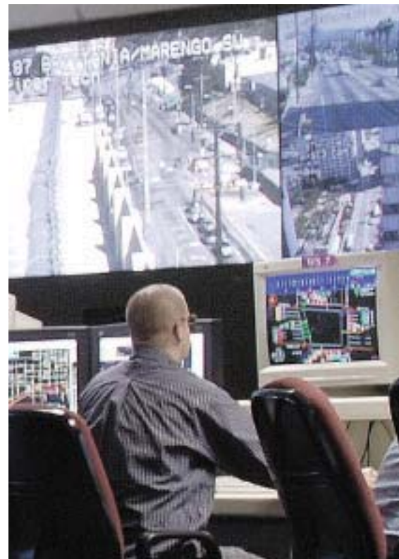
City traffic engineers monitor traffic conditions and adjust signal timing in a state-of-the-art technology center.
